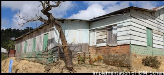
Implementation of IDMI Scheme in Mizoram.
