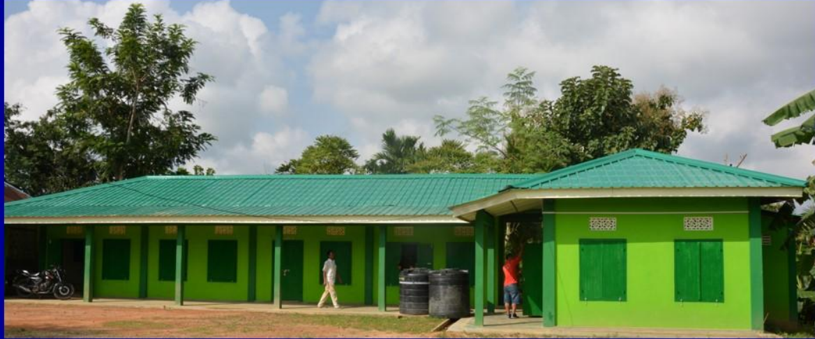
Thinghlun Adhoc Aided H/S newly constructed/strengthened under IDMI Scheme
