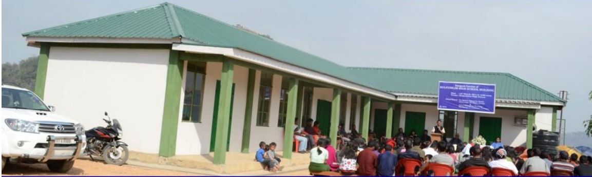
Ailawng Aided H/S newly constructed/strengthened under IDMI Scheme
