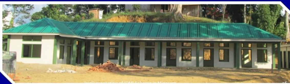
Implementation of IDMI Scheme in Mizoram.
