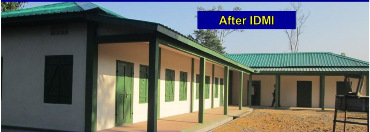
West Bunglemun Adhoc Aided H/S newly constructed/strengthened under IDMI Scheme
