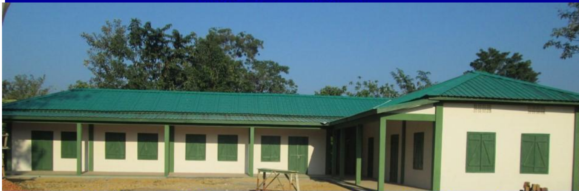
Zawlnuam HSS newly constructed/strengthened under IDMI Scheme
