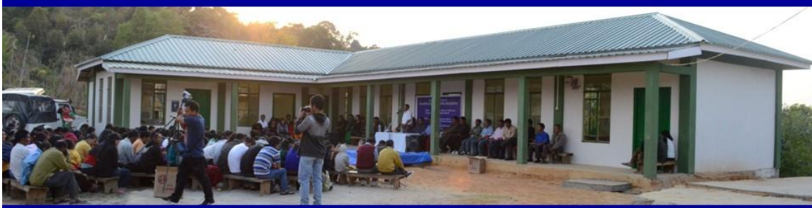
Rulpuihlum Adhoc Aided H/S newly constructed/strengthened under IDMI Scheme
