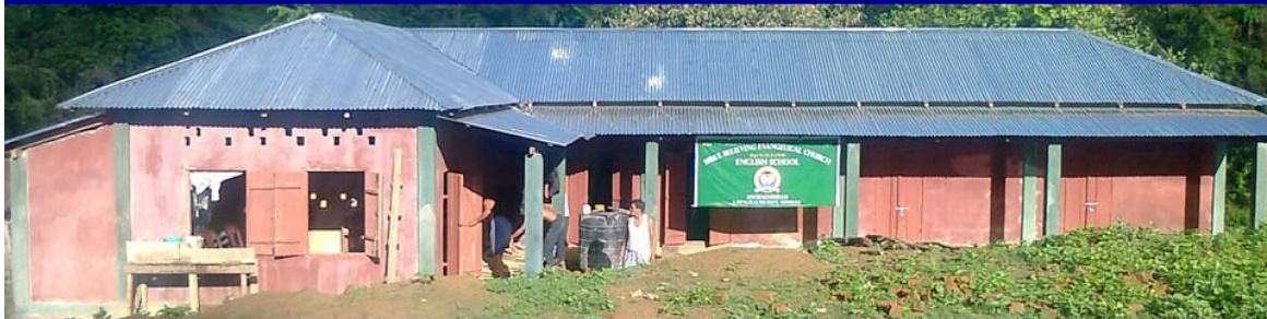
Zochachhuah English School newly constructed/strengthened under IDMI Scheme
